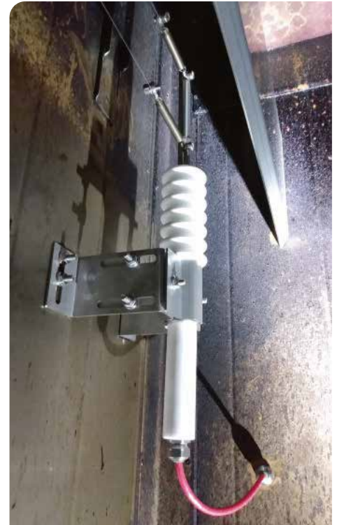
The isolators inside the smoke system are configured so that stable high voltage can be applied constantly. Photo: EBSmoke
